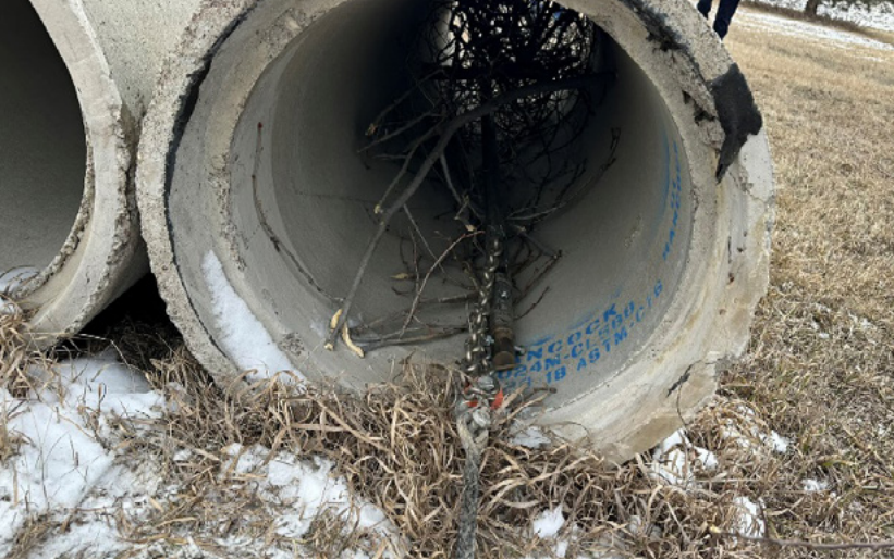
Stockpiled culvert jammed with brush
