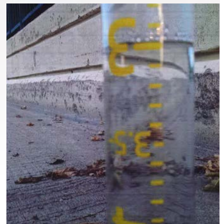
Treated bridge deck showing virtually no loss of water
