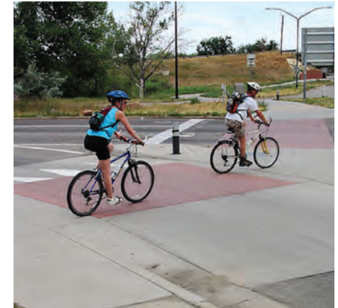
CHANNELIZED TURN LANE WITH RAISED CROSSING
