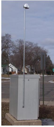
Figure 3: GPS radio antennas attached to cabinet
