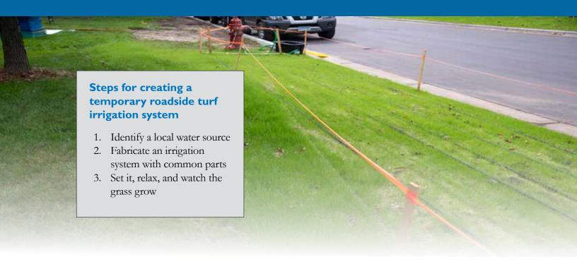
The temporary system and a control plot were installed along a portion of the project that was not watered by a permanent irrigation system. City staff monitored staff time, gallons of water, and length of time to achieve 90 percent coverage with 6-inch turf grasses.
