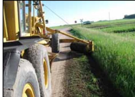
**Problem** The gravel from gravel roads or shoulders is often pushed out and down the slopes of Sibley County roads, causing rough conditions and pavement edge drop-offs. For gravel shoulders on paved bituminous highways, two motor graders were used in reclaiming operations, one with a retriever and the other to blade the gravel back onto the shoulder. This process was expensive in terms of budget and personnel, as it required two graders and operators.
