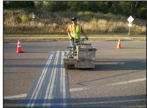
**Solution** The county installed a thermoplastic coating attained from P.K. Contracting in Troy, Michigan, to minimize or eliminate this problem on roads and trail systems.
