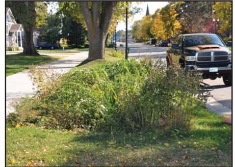
**Solution** The City of Grand Rapids began constructing modified rain gardens as part of a 2008 street reconstruction project on First Avenue Northwest. Since the rain gardens are not large enough to be used solely as infiltration basins, they are connected and allowed to discharge to the city's storm sewer system.
